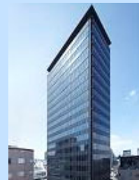
Urbannet Kanda Building Total floor space: 14,724.77 m 2
