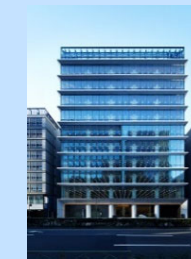
Urbannet Nihonbashi 2-chome Building Total floor space: 14,674.49 m 2
