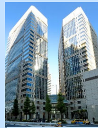
Otemachi First Square Total floor space: 143,206.98 m 2
